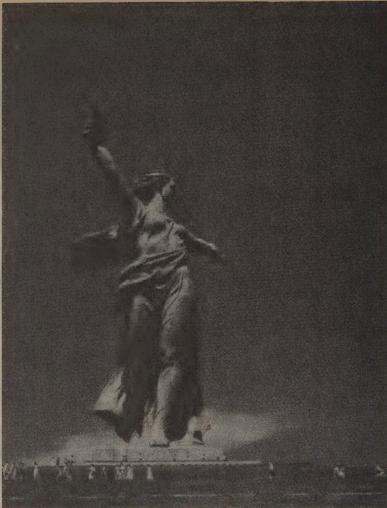
The 270-foot statue of Motherland (Volgrad) is not fixed to its pedestal, its own great weight providing the only support. The scarf blowing away behind the neck
